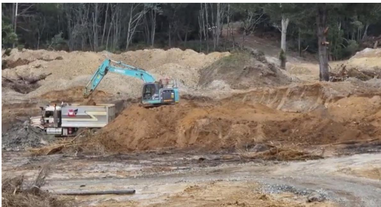
Figure 2: Excavation in the Wetlands environmental cleanup area.
